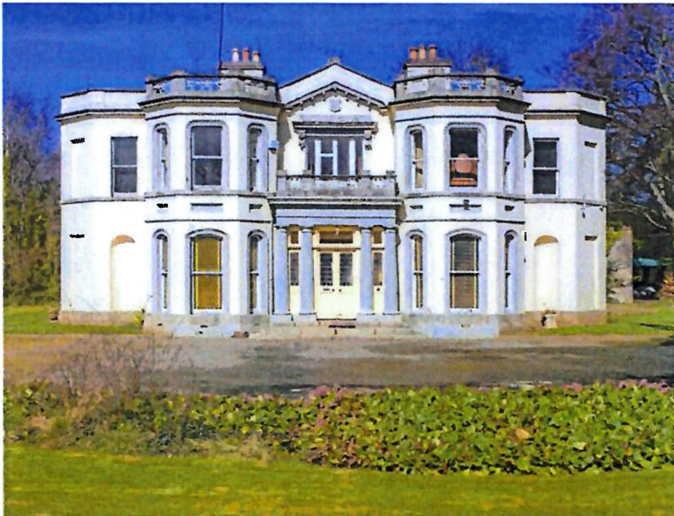
Figure 3: Image of the Front Elevation of Beauchamp House. Source: Irish Times.
